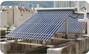
(3) The life expectancy of solar collectors is about 20-25 years and some contractors will provide product warranty depending on procurement requirements. Before replacing a faulty solar collector, its warranty shall be checked.
